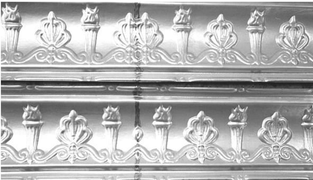
If the plaster on the walls is suitable (not too hard or not too soft) the cornice can be nailed to the wall using suitable concrete nails (25mm x 3mm fluted nails for example).
